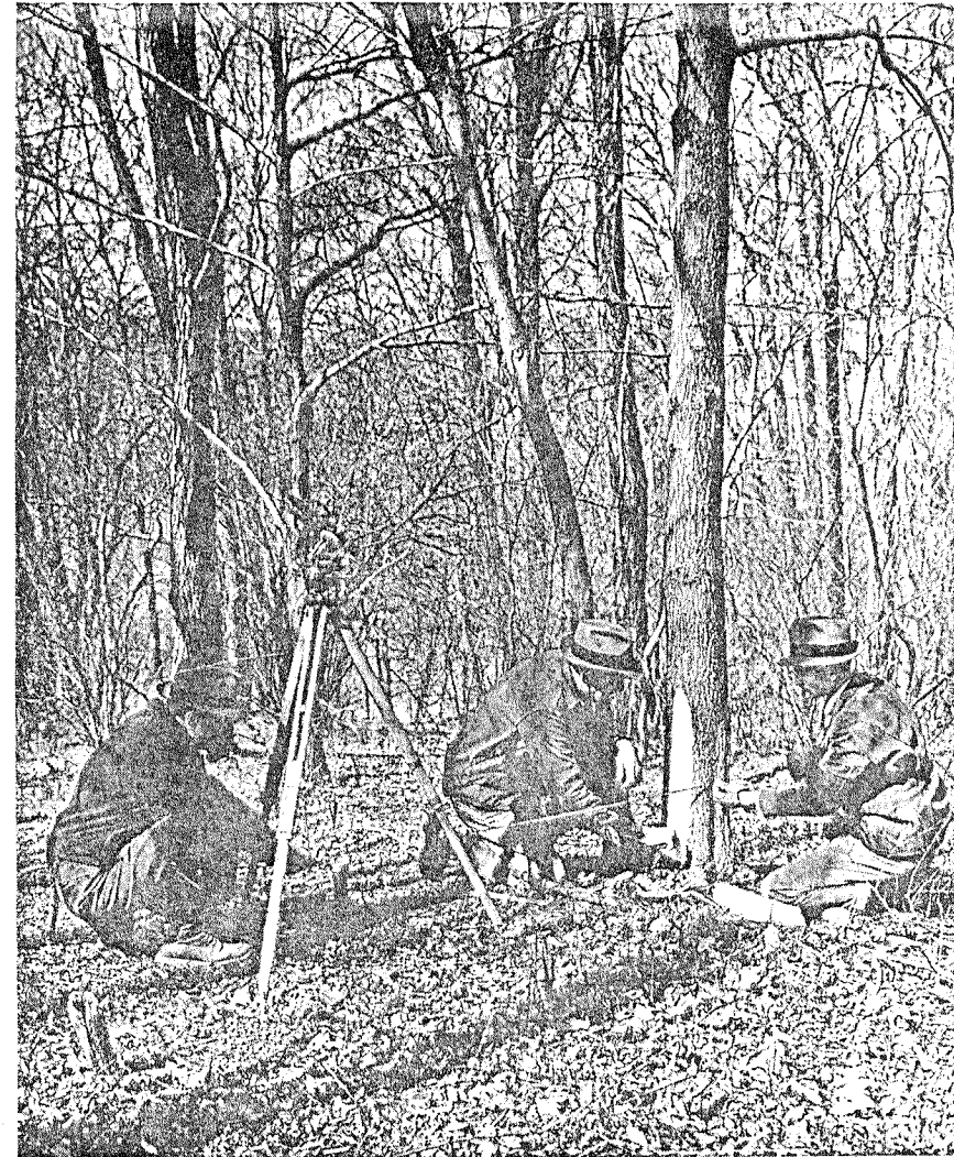
Marking a bearing tree as an accessory to a corner.
